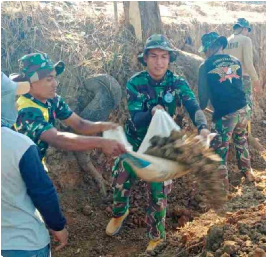
Kasdim 0811 Tuban Mayor Caj Sunarso mengecek langsung hasil plengsengan
